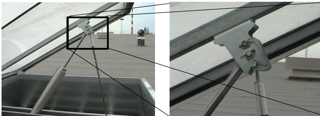
Fig. 27. Connection of actuators to the hook console.
